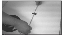
2. Temporarily adhere LEDs to back using masking or electrical tape according to layout or estimate and test to ensure evenness of illumination prior to final install.
